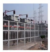
The SPGLbTBB series open rack capacitor banks are especially designed to compensate the reactive energy and power line loss in power networks outdoor for the normal load in 6-550kV power system and DC transmission, as well as special off for the load with harmonics content, permitting not only the correction of the fluctuation caused by lineal, but also the non-lineal electrical loads.
