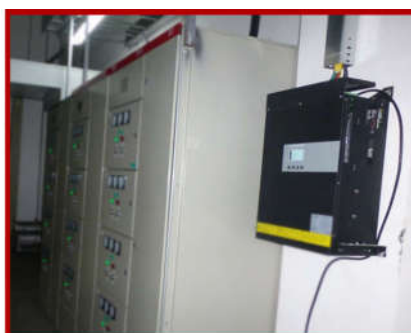
Wall mounting on site
